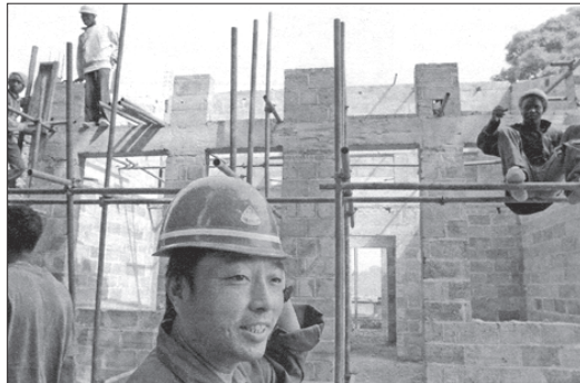
A Chinese foreman at a construction site in Guinea-Bissau. Developing countries like China, India and Brazil are strengthening economic and political relations with Africa.
