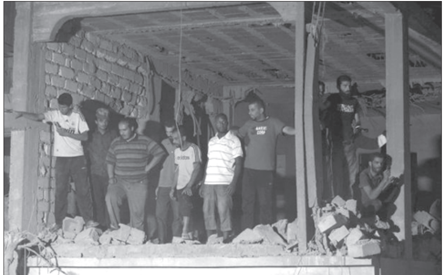
Libyans inspect the rubble of a house in Tripoli said to have been destroyed by NATO airstrikes. Almost immediately once NATO launched its Libyan operations, it was clear that an entirely new and controversial mission was under way than what was acknowledged in the debate preceding the Security Council authorisation.
