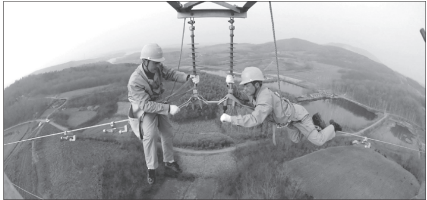
Chinese workers checking on an electricity pylon. In terms of installed capacity, China has the largest electric power system in the world.
