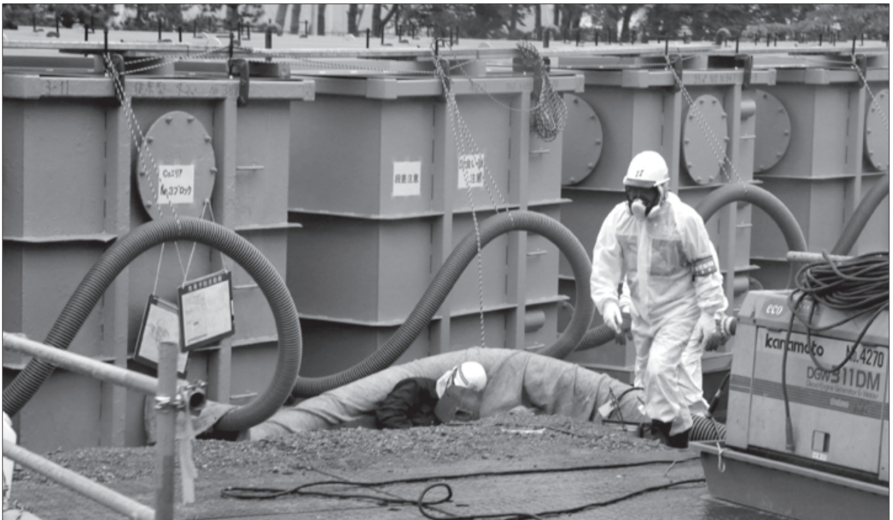
A worker walks amid water tanks at the tsunami-hit Fukushima Daiichi nuclear power plant. The continuing problems at Fukushima Daiichi during the last four years stem from skewed priorities favouring the nuclear industry.
