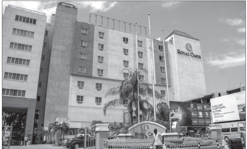
As part of the reconstruction programme in Haiti after the 2010 earthquake, a fund set up by two former US presidents invested in the Royal Oasis (pic), a deluxe hotel in the heart of Port-au-Prince, where people were suffering from extreme hardship.
