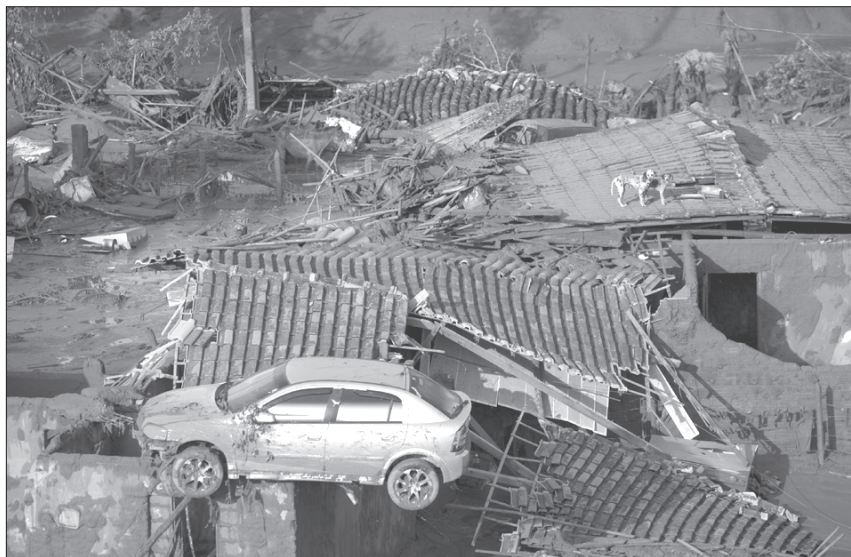
The collapse of a dam at a Brazilian mine on 5 November buried the town of Bento Rodrigues under contaminated mud.
