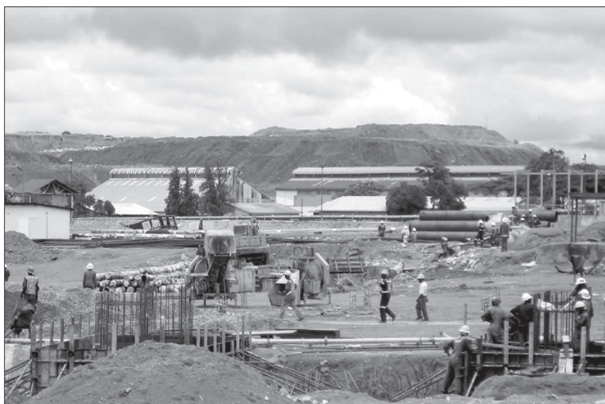
A copper smelter under construction in Chingola, Zambia. Zambia has suffered substantial losses in terms of foregone mining tax revenue partly due to corporate tax avoidance.
