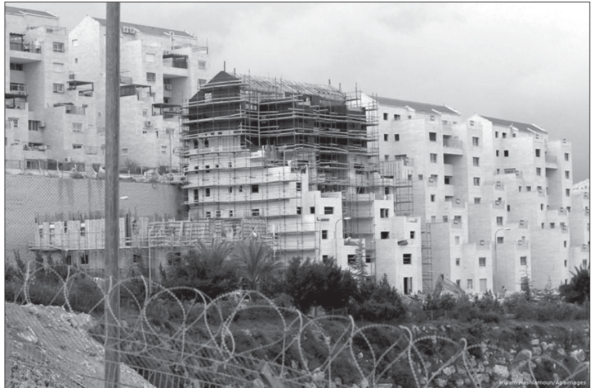
Construction work on a Jewish settlement in the occupied West Bank. In 2017 Israel intensified the expansion of settlements and housing units in the West Bank.
