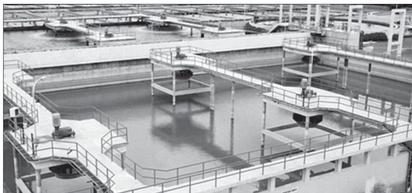
Concerns have been raised over the potential role of sewage treatment plants as breeding grounds for AMR.
