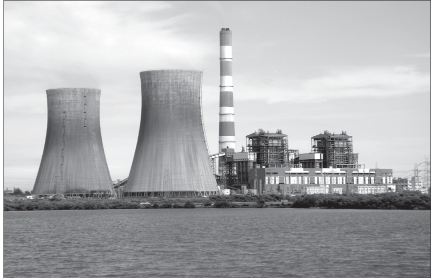
A coal-fired power plant in India. Some 47% of the country's primary energy supply and 71% of electricity generation are dependent on coal.
