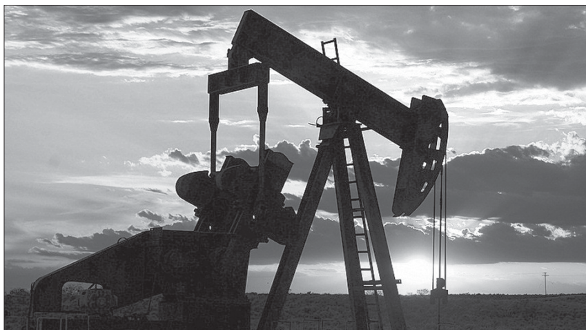
An oil pump jack in operation in Texas. President Biden is being called upon to reject two massive oil export terminal projects proposed for the Texas Gulf Coast.
