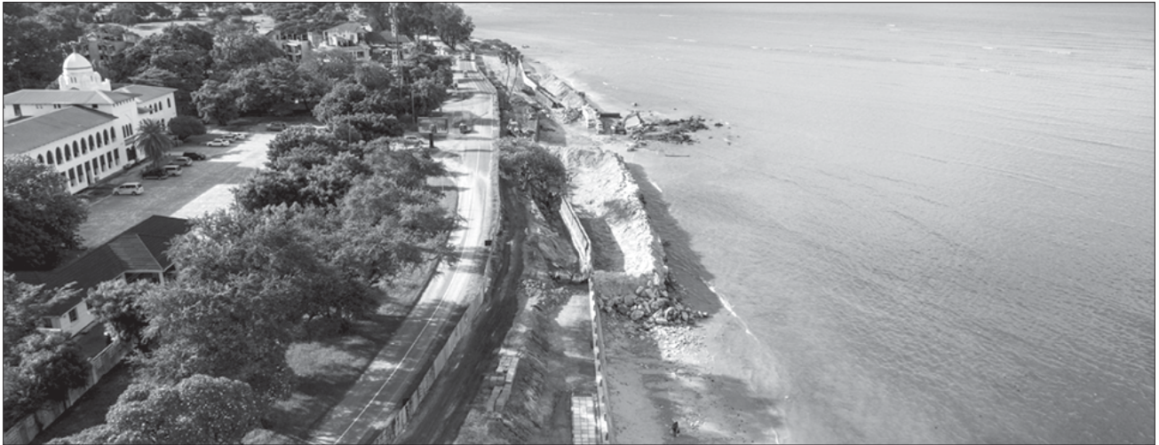
A seawall project in Tanzania to protect against rising sea levels sparked by climate change. The Glasgow conference launched a work programme on the global goal on adaptation to climate change.
