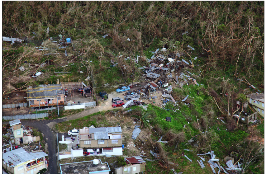
A scene of the devastation wrought by Hurricane Maria in Puerto Rico in 2017. Hurricanes in the Caribbean are becoming more extreme due to global warming.
