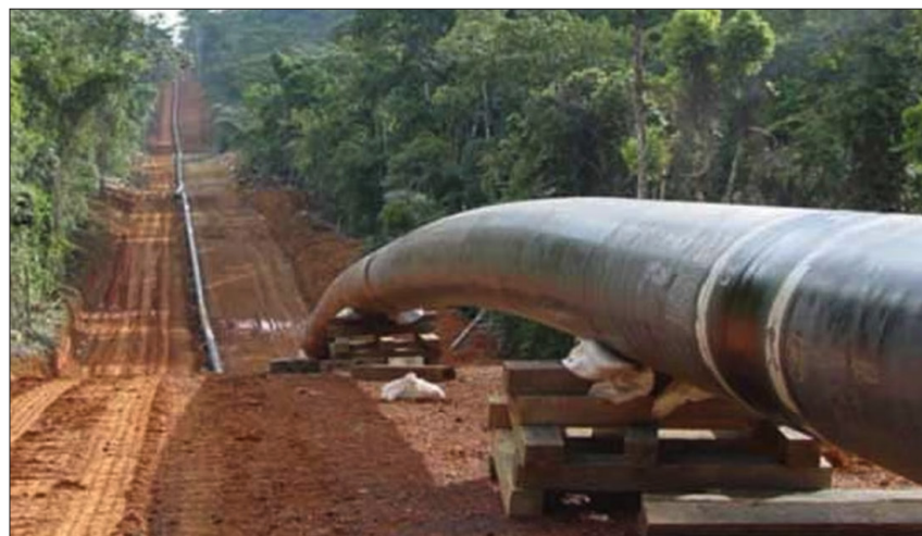
The East African oil pipeline being built by French energy giant Total in Uganda and Tanzania is mainly to serve Europe.
