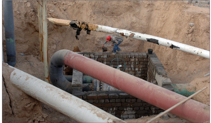
Repair works on an oil pipeline at the Al Fatah bridge in Iraq in 2006. The US invasion enabled multinational companies to once again exploit Iraqi oil, ensuring Western energy security.
