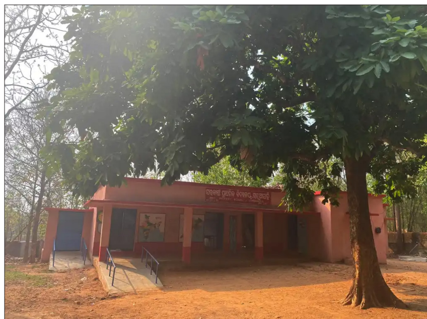
This government primary school located deep in the interiors of Mayurbhanj district is one of about 1,500 schools in Odisha where the MLE programme is being implemented.
