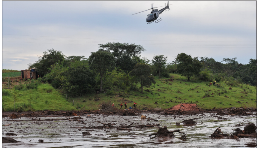
In January 2019, a mining dam owned by Brazilian company Vale collapsed in the municipality of Brumadinho, sending 12 million cubic metres of mining waste down the Ferro-Carvão River.
